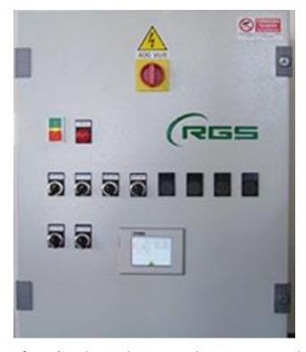
We can offer compatible software's and control systems making processes work Fully Automatically, Semi Automatically and Manual Mode. Control box is equipped with all standard parts including PLC, Transformers, Thermal overload, Switches and so on.
